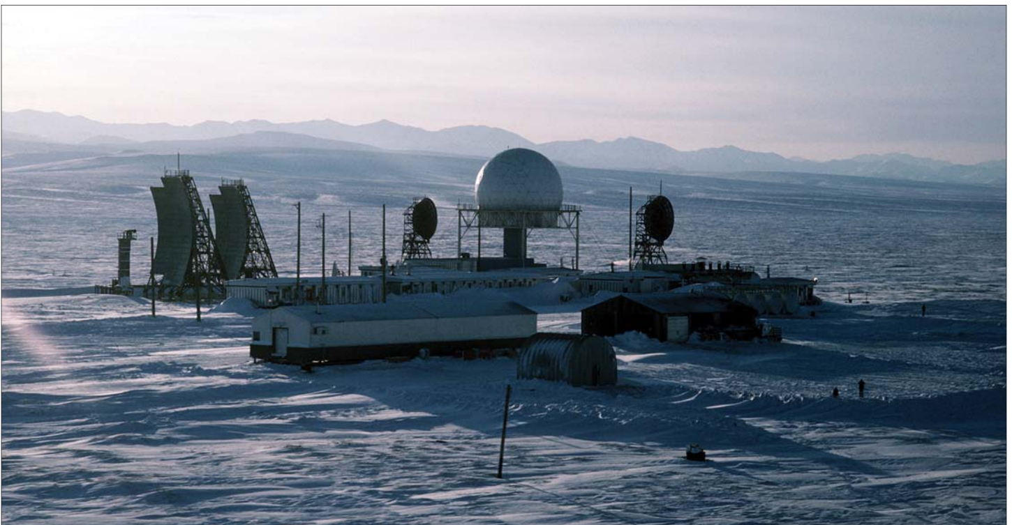
Above, the now-defunct radar station LIZ-2 at Point Lay was one of 30 stations under U.S. Air Force control on the Distant Early Warning Line that ran approximately 3,600 miles from Alaska across Northern Canada to Greenland. The curved White Alice antennae are shown on the left. LIZ-2 was commissioned in 1955 and dismantled in 1989. Photo by Air Force Tech. Sgt. Donald L. Wetterman
