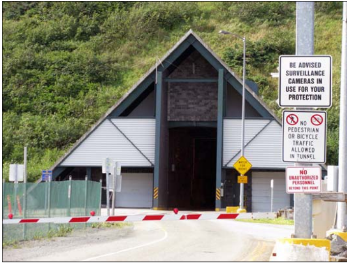
The Whittier Tunnel, above, a combined one-way road and railway tunnel. Photo by Flickr user Arthur Chapman, and Audrey Bendus
